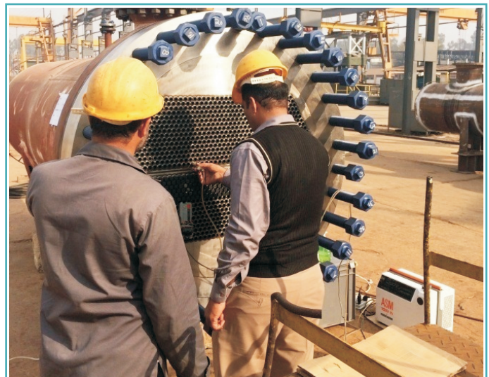
Helium Mass Spectrometry Testing of Heat Exchanger being done for M/s at DESCON Engineering Ltd Lahore
